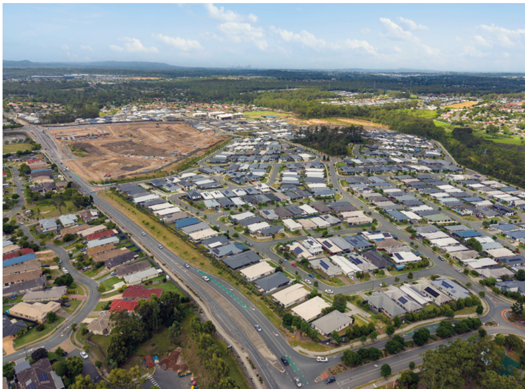
Woodlinks, showing bulk earthworks under way for Stages 25-27 and the commercial site.
